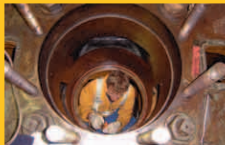
Ballance Maintenance Technician Barry Jordan had to work in confined spaces
