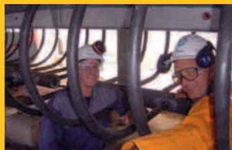
Projects engineer, John Carley (left) and General Manager Operations, Warwick de Vere, inspect the welding project
