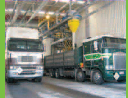
Trucks loading at Timaru on the first day of despatching from the upgraded plant
